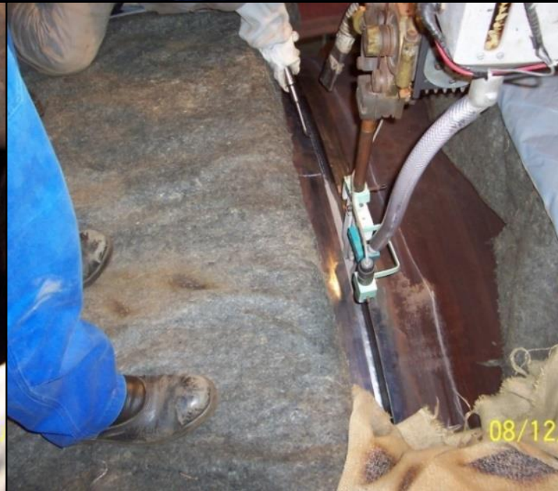
SUBMERGED ARC WELDING (SAW) NARROW GAP TECHNIQUE
